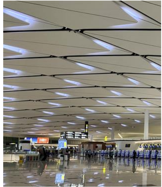
Building ceiling – interior
